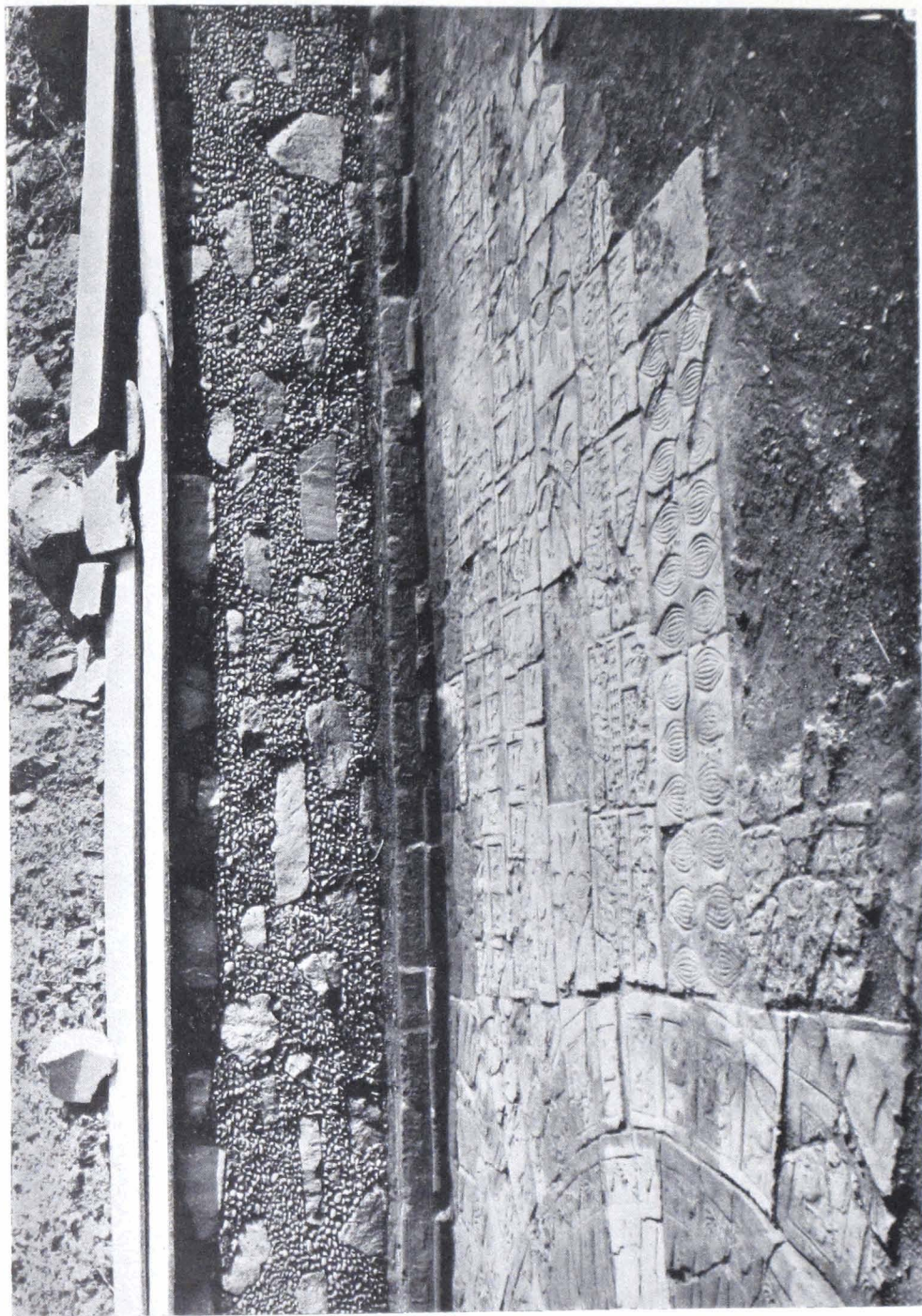
HARWAN : WALL OF APSIDAL TEMPLE IN DIAPER-PEBBLE STYLE WITH PORTION OF TILE-PAVEMENT.
